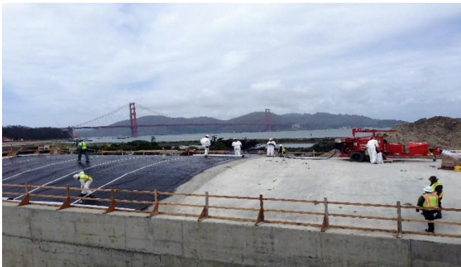
Figure 1. Positive side Waterproofing
