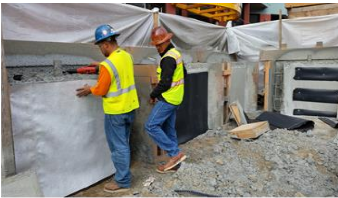
Figure 8. Installation of the outer fleece reinforced HDPE sheet.
