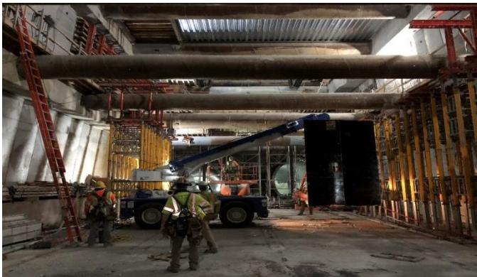
Figure 12. Central Subway top down construction
