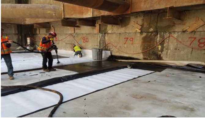
Figure 6. Field application of polymer rubber gel composite waterproofing system
