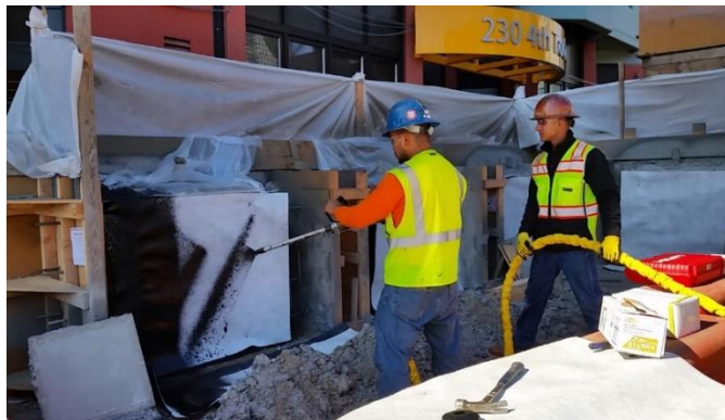
Figure 9. Spray application of PRG on fleece reinforced HDPE.
